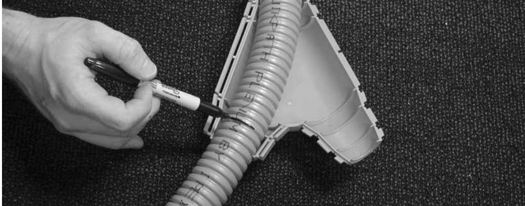
Figure 2: Determine Size of Section to be Removed
